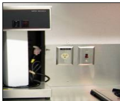
1 Interior Outlet on Lighted Switch for Coffee Maker
